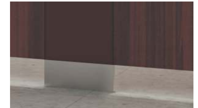
SS Shoe Box Up - 12 mm compact board
