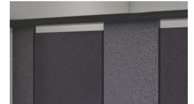
Powder coated aluminum Top rail
